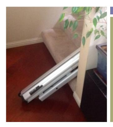
Why is the stair lift in this picture not up against the wall? In this case, the unit would have caused a trip hazard at the top of the stairs, so it needed to be installed on the right side
